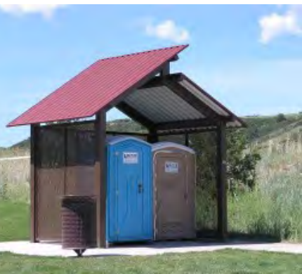
Seasonal Restroom with Screen
