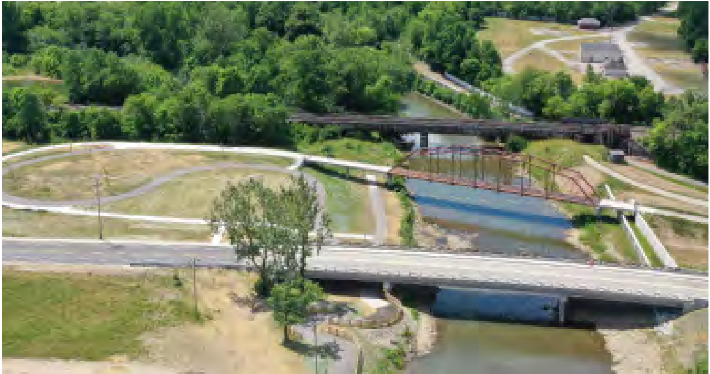
Kitselman Trailhead – Refurbished INDOT bridge for pedestrian use (Kitselman Trail – Muncie, IN)
